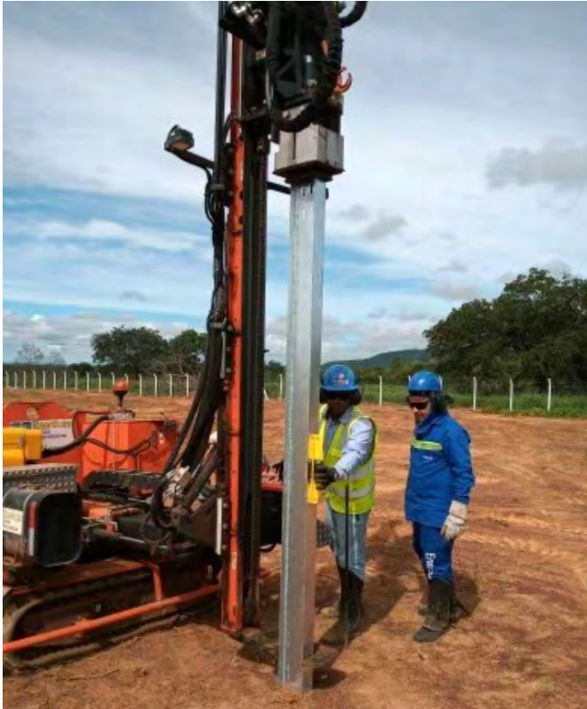
Figure 5-4A Ramming posts
