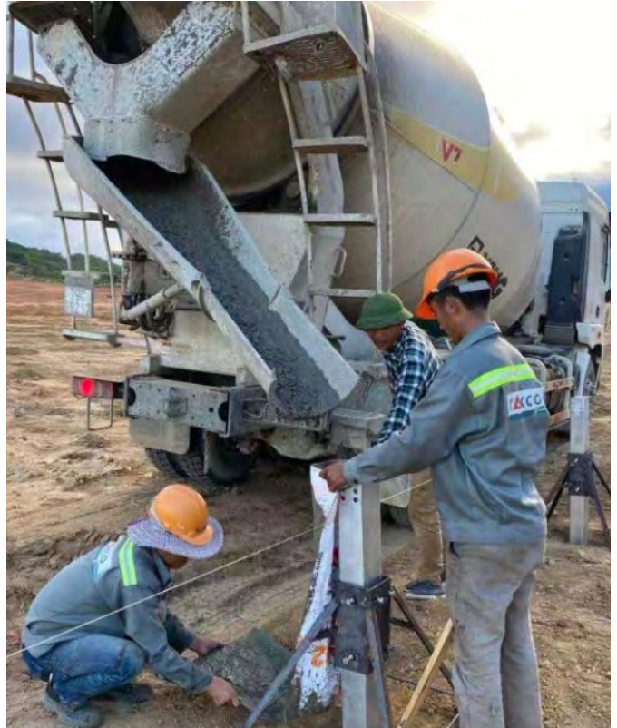
Figure 5-4B filling concrete piles
