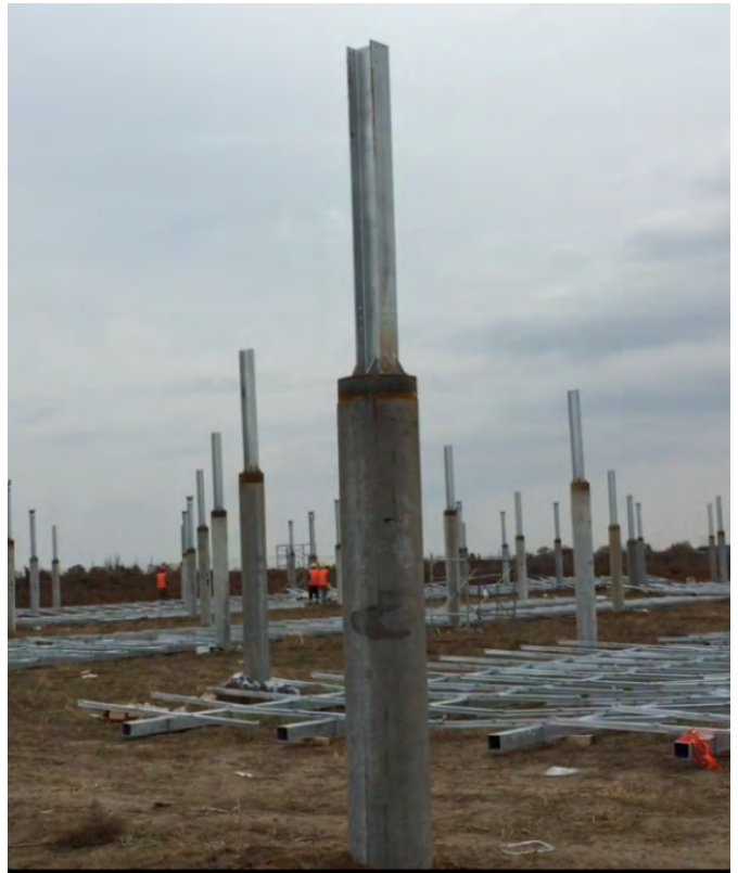
Figure 5.8B Welded steel post on top of PHC pile
