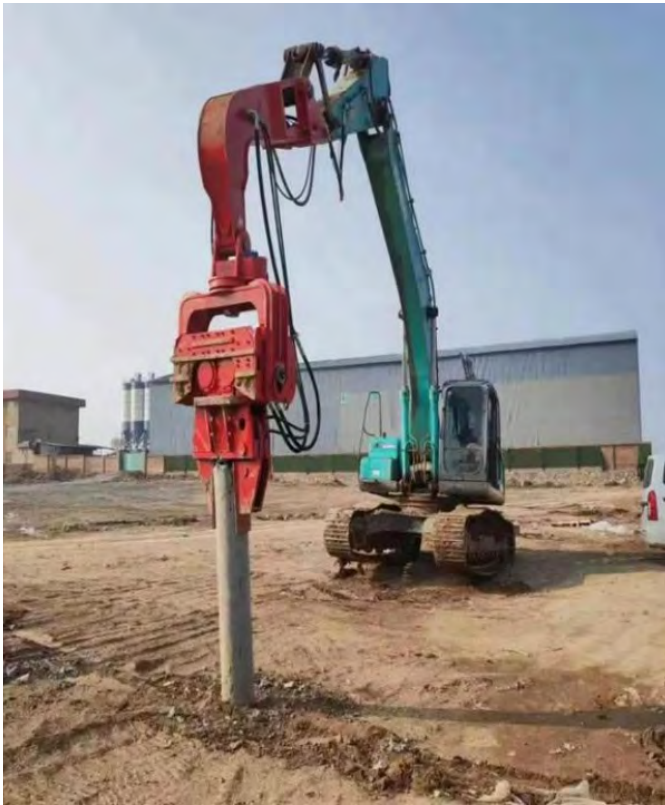
Figure 5.8A PHC pile driving construction
